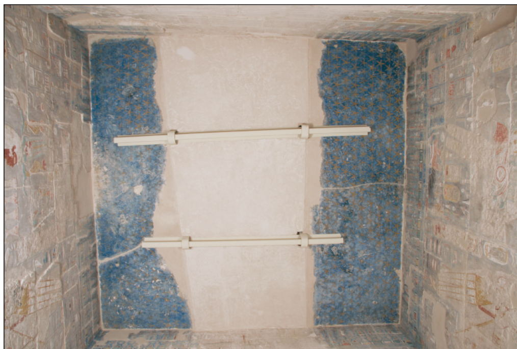
Fig. 3. Southern Chamber of Amun-Re. Ceiling after restoration (Photo M. Jawornicki)
